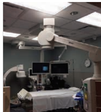
Clockwise from top: Edward Hospital, Naperville, Illinois > HTC's Accu-Mount Support Systems safely and easily attach medical equipment to an overhead building structure. > Healthcare Technology Corporation supplied a total of eight mount supports for two ORs.
